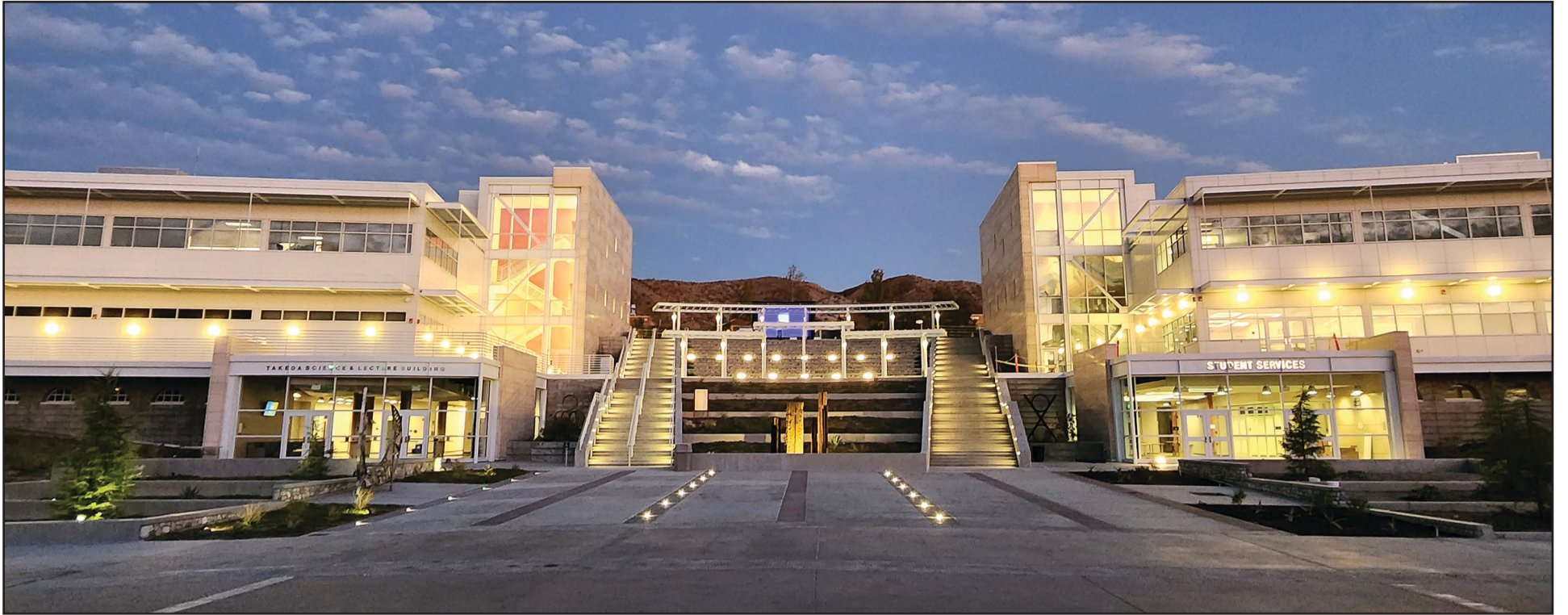
Major construction has been completed on the Student Services/Learning Resources Center (right), whose design mirrors the Takeda Science Center (left) at the Canyon Country campus.
